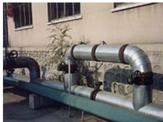
Ultrasonic descaling & anti-scaling for air compressor in refinery.
