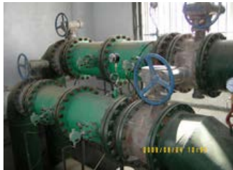
Ultrasonic descaling & anti-scaling for H-type steel workshop in steel factory.
