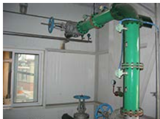
Ultrasonic descaling & anti-scaling for sewage pipeline in treatment plant.
